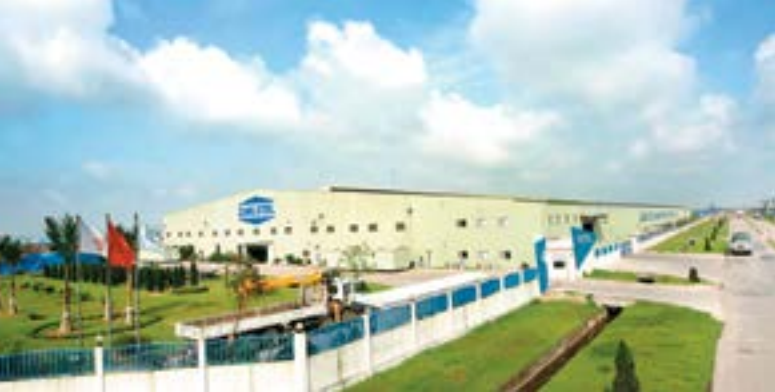
Hanoi Plant Total Area – 41,200 sq.m Fabrication Capacity, 5,000 MT per month
